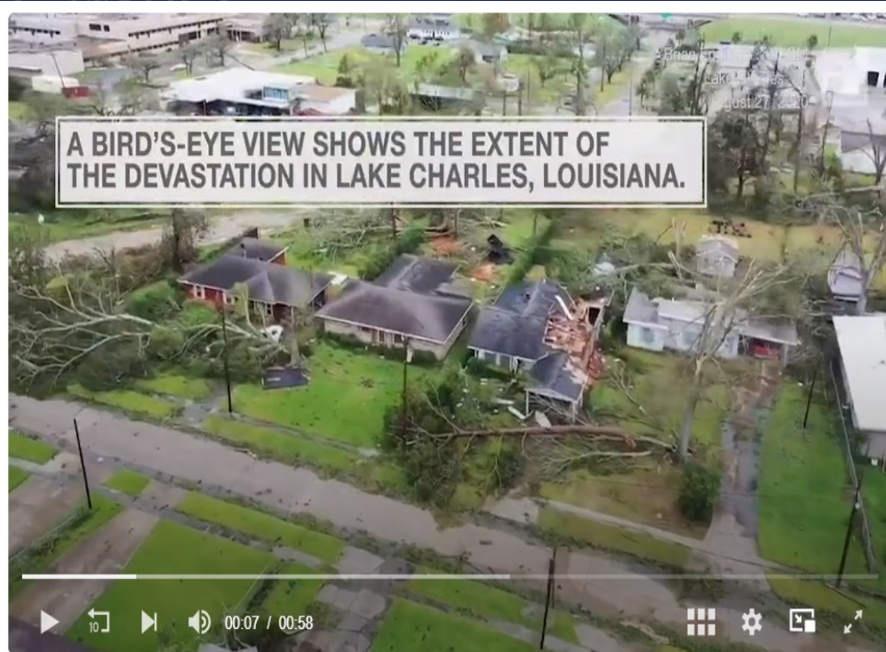
Aerials Show Dramatic Extent of Hurricane Laura Damage in Lake Charles
